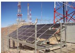
The system is capable of providing telecommunications equipment with power, autonomously and independently of the mains electricity. For this purpose, a photovoltaic solar power system has been provided with a high-capacity storage system based on jellified and sealed lead electrolyte batteries.
