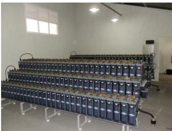
Mature Batteries (Lead, Ni-Cd, Lithium) are still expensive nowadays as a mass electrical storage for long periods of regulation of renewable production. Nonetheless the right sizing criteria of renewable resource, battery capacity and the correct dispatching strategy, together with the optimum gen set operation point might result in a cost competitive levelised cost of energy as compared to plain diesel based forms of
